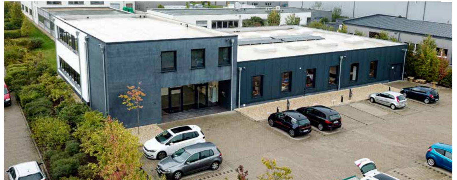
Our premises in Meckenheim
